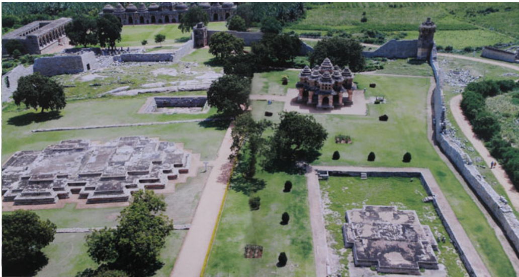
Fig. 8 Aerial view of the Zenana Enclosure
