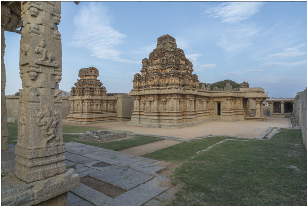
Fig. 4 Hazara Rama temple in the Royal Centre
